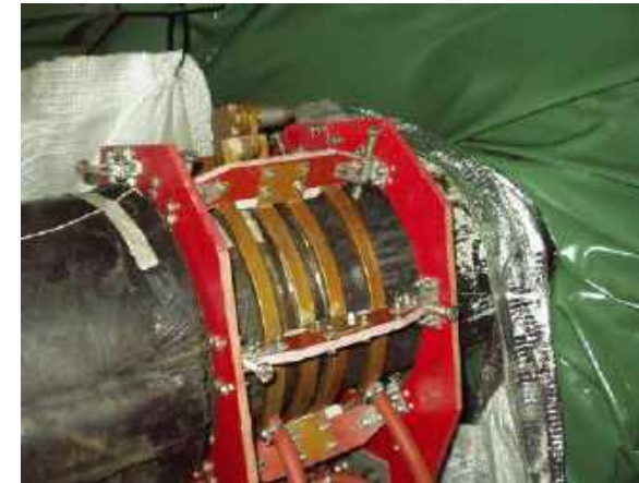
Gambar 10.3 HF local heat treatment(TWI, 2018)
